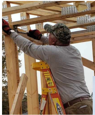
A crew from Hope's Helping Hands ( Leslie & Doug Daniel; Rod & Laurie Christman) spent a Saturday on the east side of Allentown installing ceiling joists for a Habitat for Humanity Build. The beams above the group, in the picture to the left, were installed by the group.
